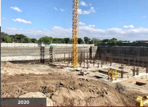
Arbor Lanes Phase 3 Block 4_5 (Arca South, Taguig City)
