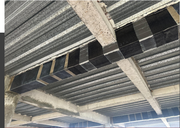
Carbon Fiber Installation
