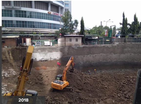
One Filinvest Building (San Antonio, Pasig City)
