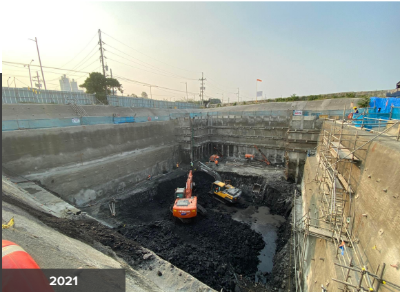
Metro Manila Subway Project Launching Shaft (Ugong, Valenzuela)
