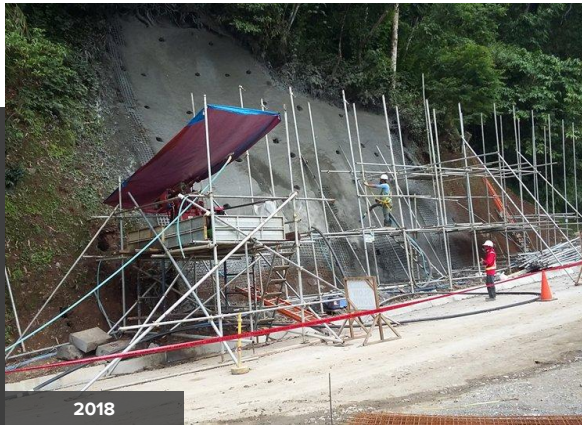
Angat Water Transmission Improvement Project (Norzagaray, Bulacan)
