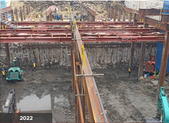
Metro Manila Subway Project (North Avenue Station)
