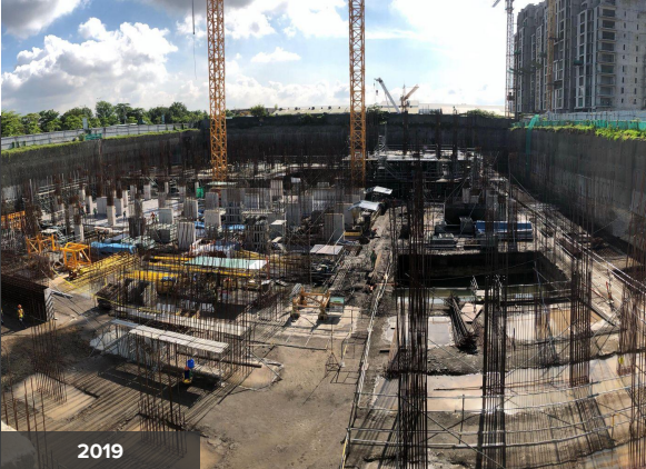
Park Cascades Phase 1_2 (Arca South, Taguig City)
