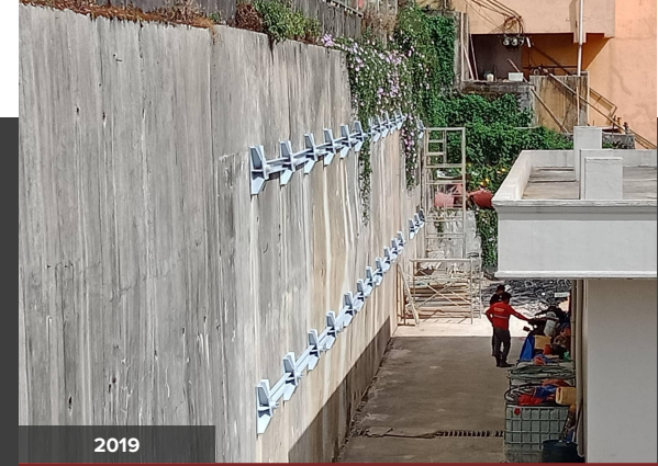
PLDT Baguio Retaining Wall Rehabilitation (Naguillan, Baguio City)
