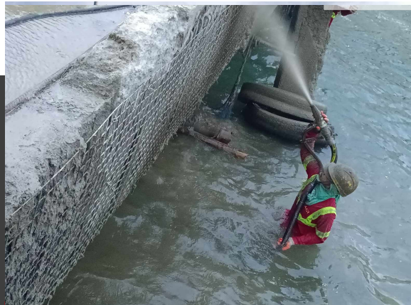
TSP Marine Pier Repair
